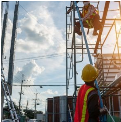
Construction Workers Tips
